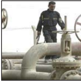
Pipeline Protection Patrolling
